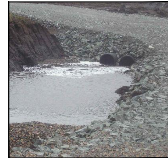
TYPICAL UNDER TRACK DRAINAGE
