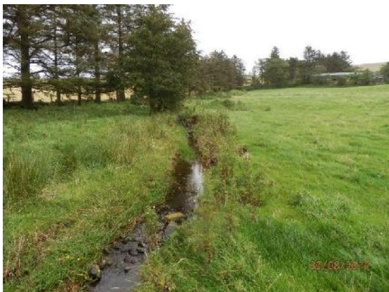
Plate 8.9: Glenarm tributary 1 culvert
