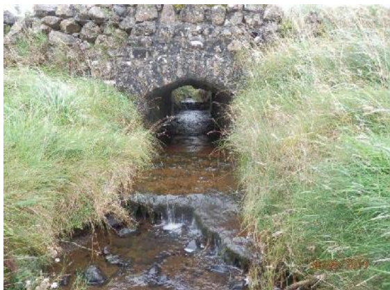
Plate 8.11: Glenarm tributary 2 - culvert
